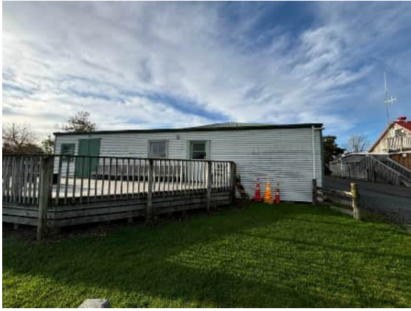
Figure 18: Southwest (rear) elevation.
