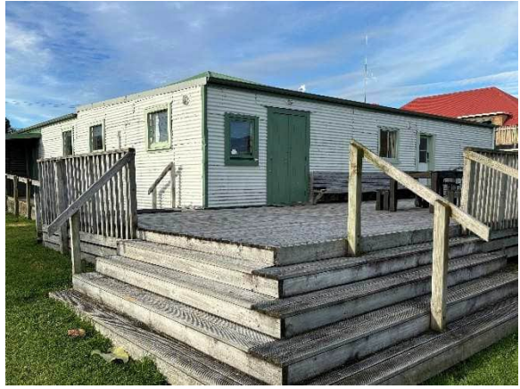
Figure 19: Southwest (rear) elevation.
